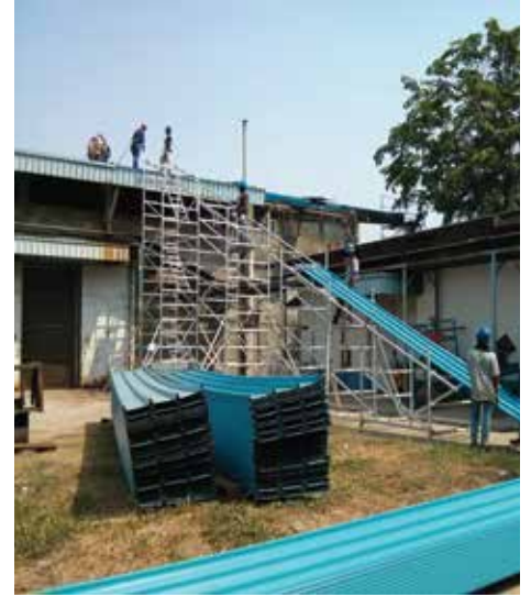
Roof Material Access
