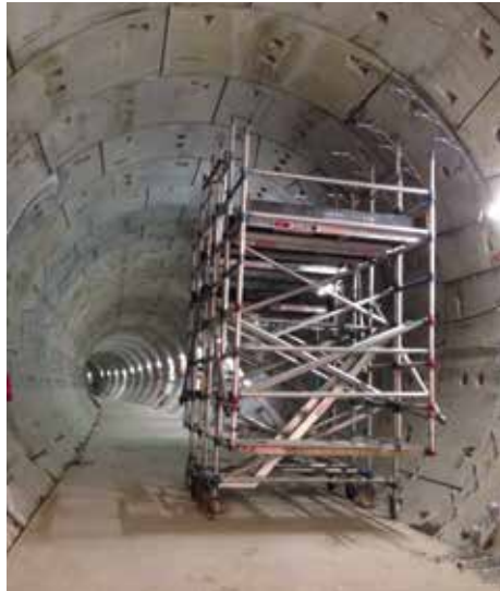
Tunnel Mobile Scaffold
